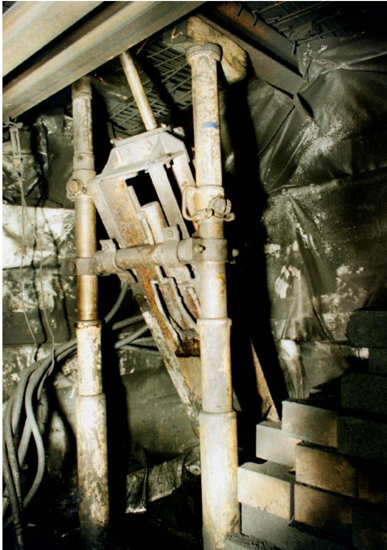
Figure 9.3 Machine de forage transversal
