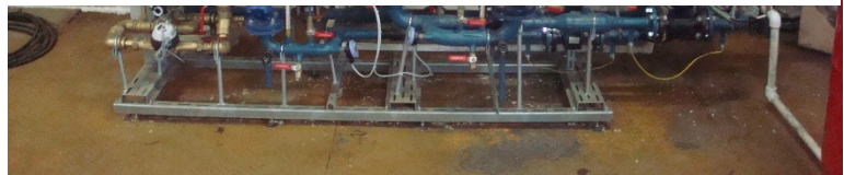
Photo I.16 Automated Individual Heat-Regulating Unit
