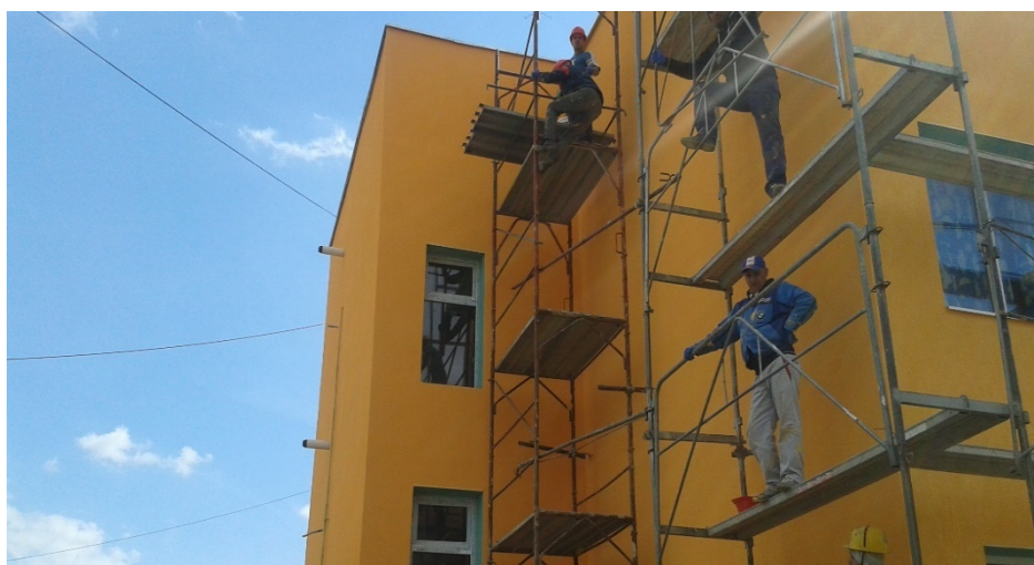
Photo I.13 Vulcan Kindergarten during Thermal Rehabilitation
