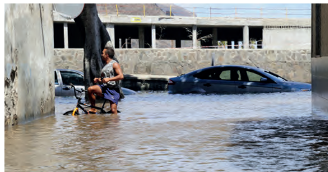
In 2011, high tide flooded the San Andres neighbourhood in Canary Islands, Spain – a consequence of rising sea levels
