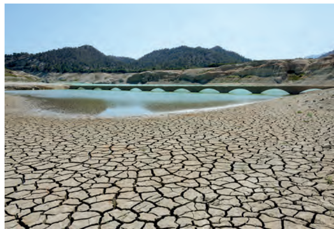
Cracks in river bottom in a water basin in Spain. Climate change will lead to an increased frequency of droughts Credit: Shutterstock/Geir Stene-Larsen
