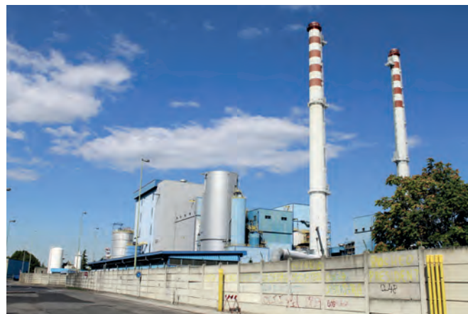
Waste to energy plant in Lombardy, Italy
