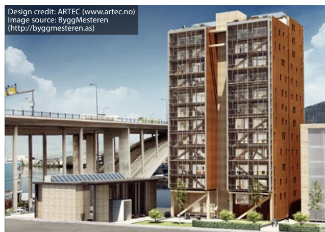
Figure 26: Verdens Høyeste trehus is a 14 storey wood apartment building being developed outside Bergen, Norway
