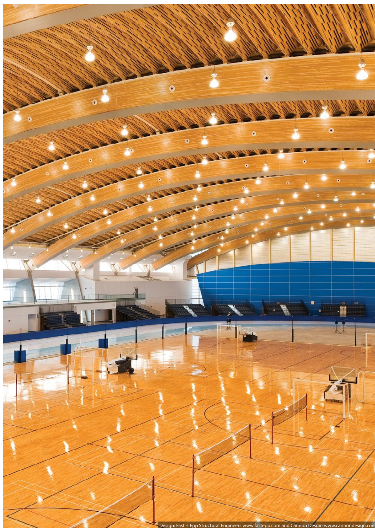
Figure 16: Innovative wood roof structure to the Richmond Olympic Oval, Canada
