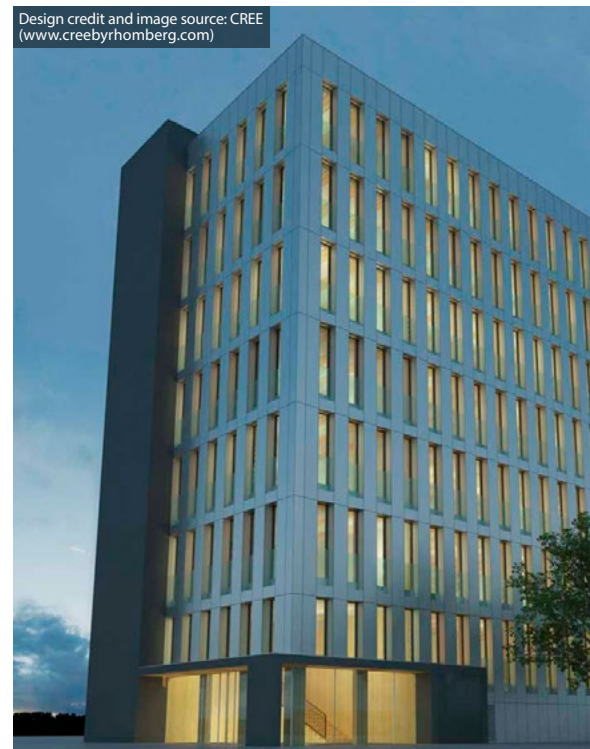
Figure 28: Life Cycle Tower (LCT) is a 10 storey wood office building in Austria
