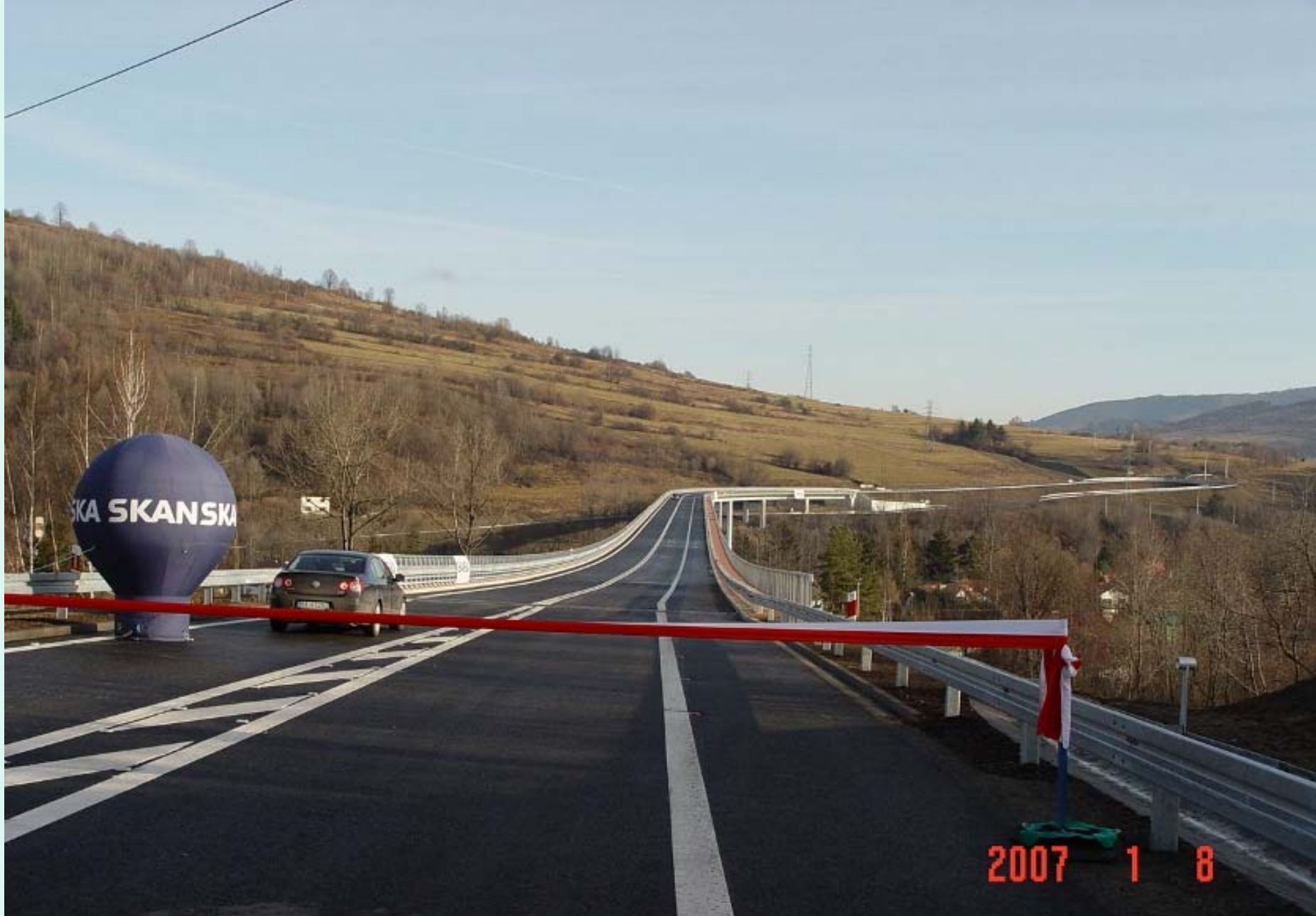
Opening for traffic the S-69 single carriageway expressway in Polish section of Corridor VI (Żywiec – Zwardoń).
