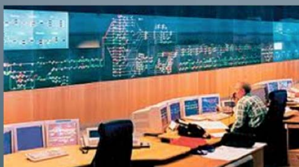
Train Control Center
