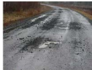
Freeze-thaw damage
