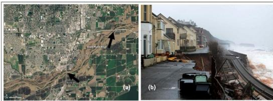
Fig. 7.9 Weather related damages to transport infrastructure. (a) Many roads, including sections of the US Highway 34 (black arrows) were washed away by the floods of South Platte River, in Colorado (USA) in mid-September 2013 ( http://landsat.visibleearth.nasa.gov/view.php?id=82090 ) (b) Damaged rail track from storm surge and waves along the Dawlish seafront, South-eastern England in February 2014 (photograph, Toby Melville/Reuters).
