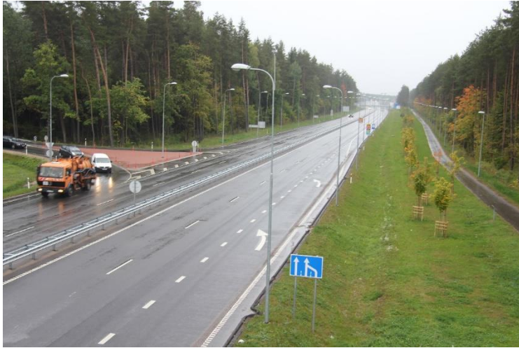
Vilnius southern bypass (5,77 km)
