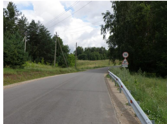
Paving of gravel roads (737 km)
