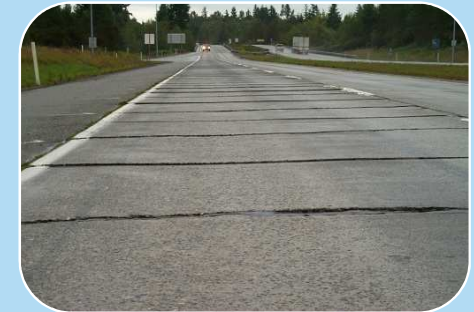
Concrete Faulting
