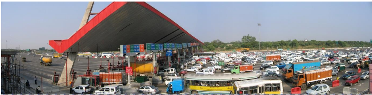
Figure 3.4: Installation of a toll plaza for a manual toll collection system
