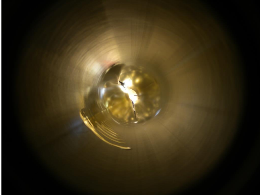
Figure 7-6: Cylinder 10 – View of the blown up area from inside
