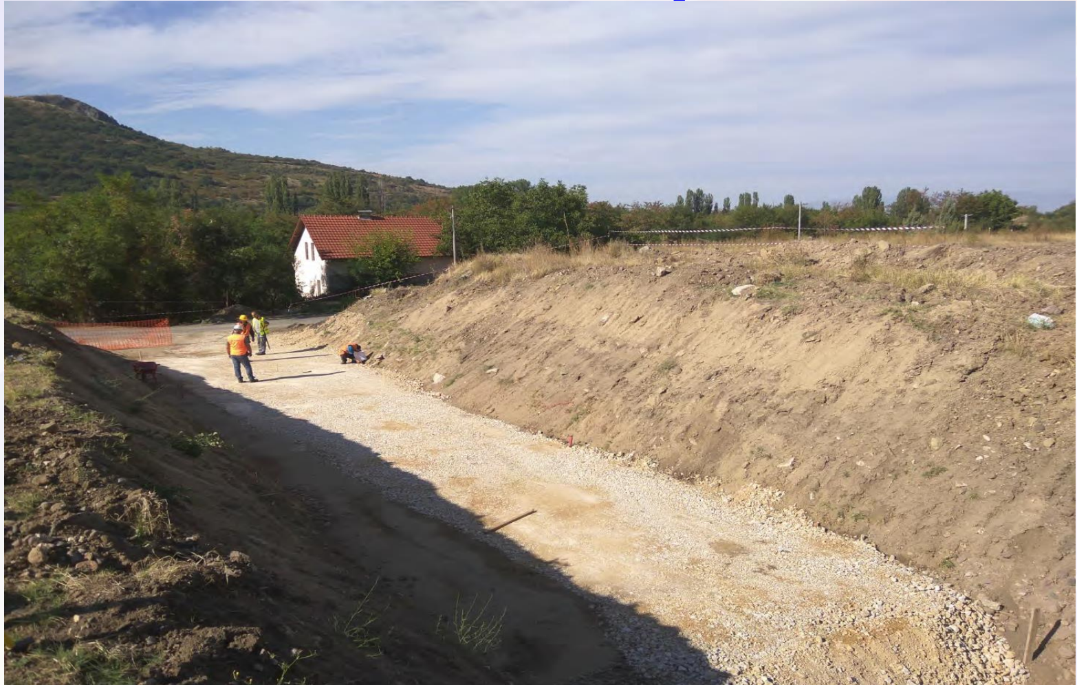
Culvert CU74 km 30+821
